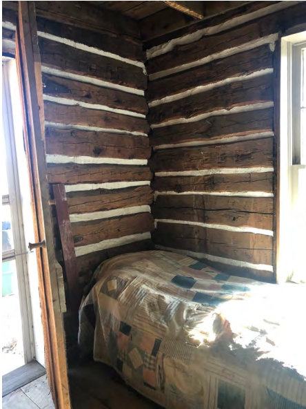
The Baugh Homestead was built as a log cabin, evidence of which you can still see in the walls, in the mid-19th century.
